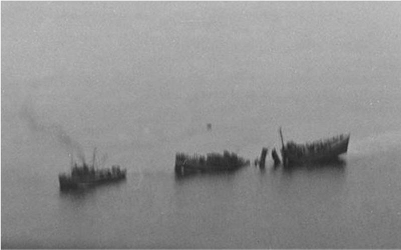
YP-346 with the *Tucker* (DD-374) under tow at Espiritu Santo, New Hebrides, on 3 August 1942. The destroyer had struck a mine while turning from Bruat Channel into Segond Channel, breaking her keel.
